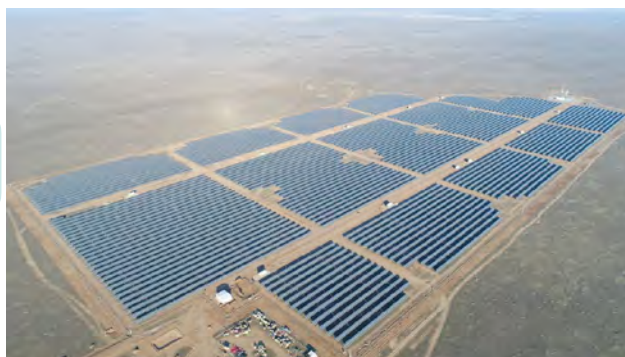
Maloderbetovskaya Solar Facility, Kalmyk Republic
